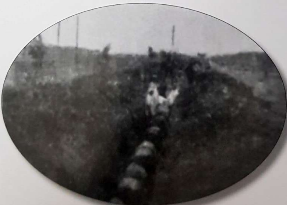
New Sind, Oct 1959, Water supply lines being laid
