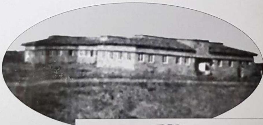
Office Building (Then)
