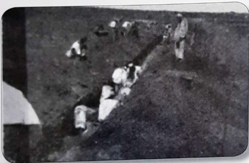
New Sind, Oct 1959, Water supply lines being laid.
