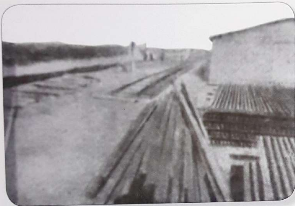
Railway lines being laid
