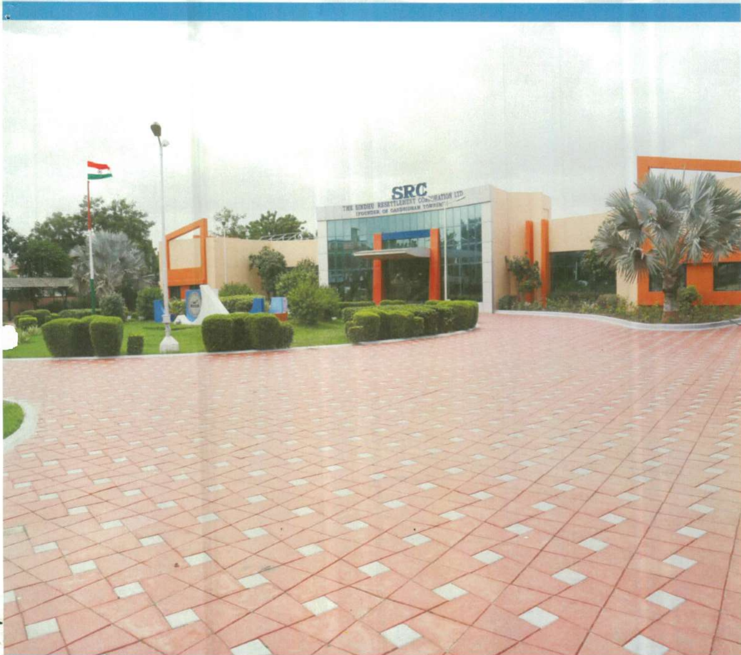
SRC AO Building at Adipur (Kutch)
