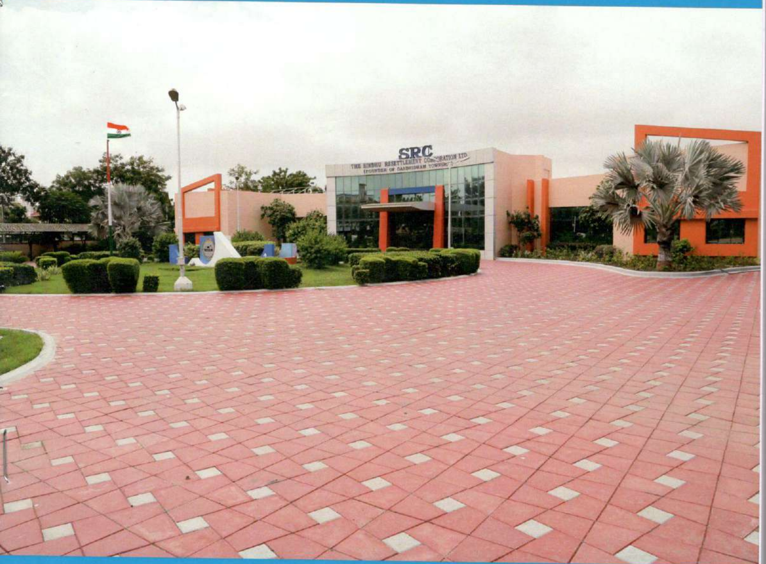
SRC AO Building at Adipur (Kutch)
