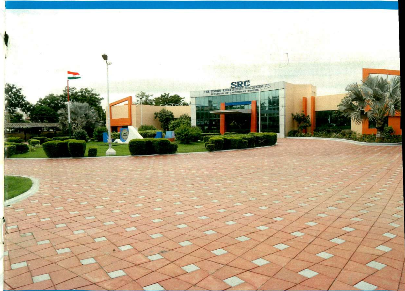
SRC AO Building at Adipur (Kutch)
