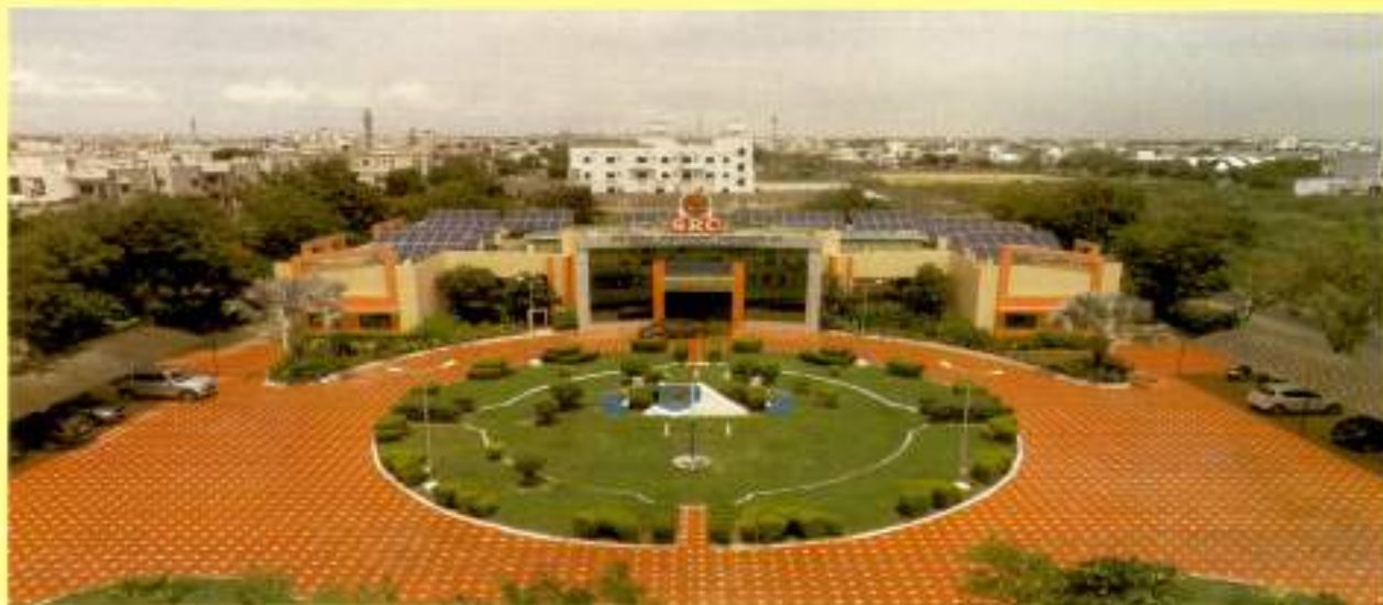
Solar Panels on Roof Top of SRC AO Building
